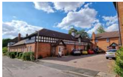
Newport Lodge Stables
