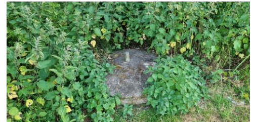
Thorpe Road Spigot Mortar
